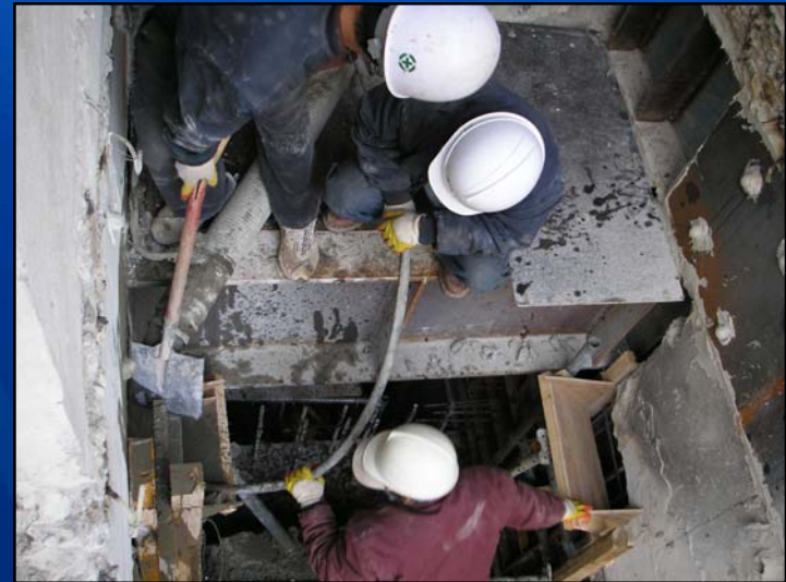
② Filling Concrete
