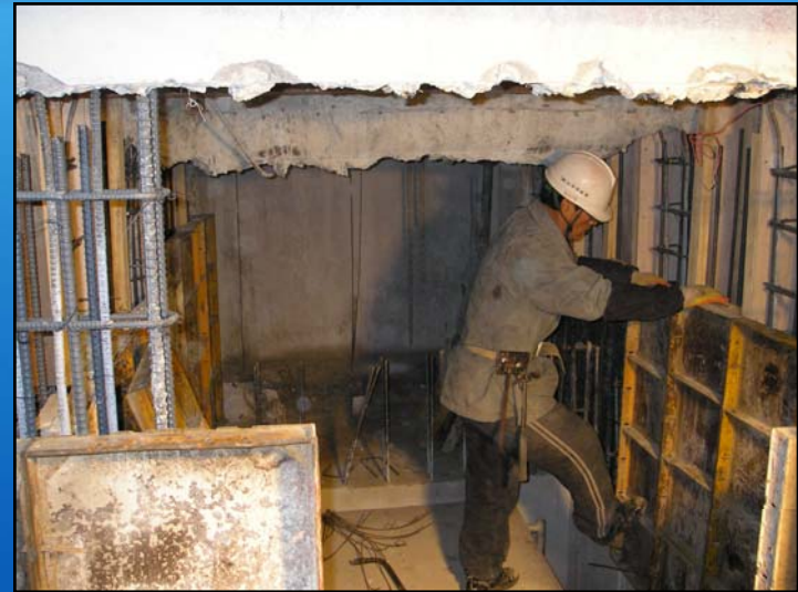
① Assembling Steel Mold
